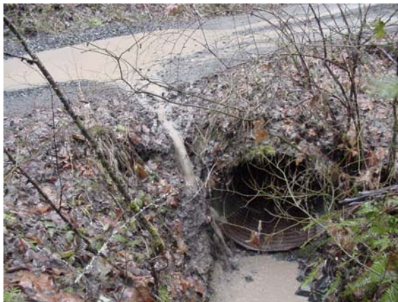
Fig 46. Sediment flowing directly into Spring Creek, tributary of East Fork Williams Creek
