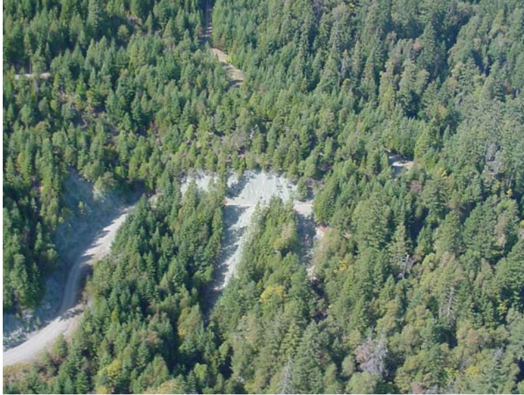
Fig 2. Aerial photo of landslide area on upper Rock Creek taken after BLM used hydroseeding techniques on the landslide to slow the erosion process. Photo by C.Rogers
