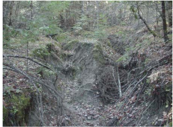
Fig 48. Gully erosion along Spring Creek Drive where erosion has cut 7 feet deep
