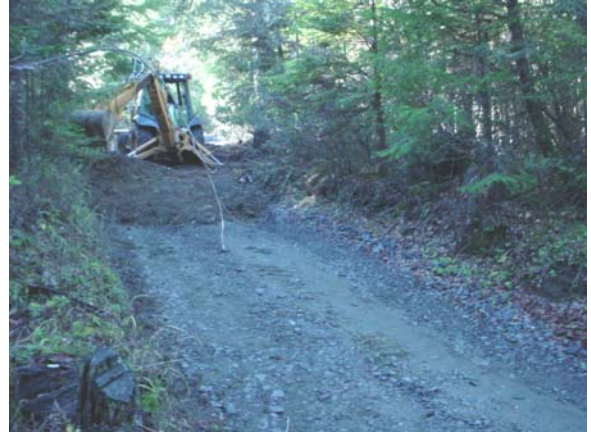
Fig 53. Backhoe fills in the road ditches
