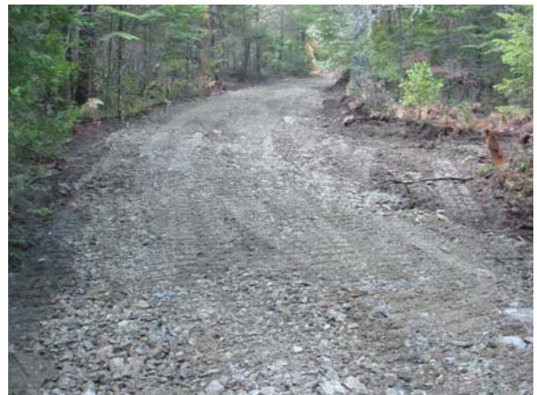
Fig 55. Completed section of road with outsloping and packed rock
