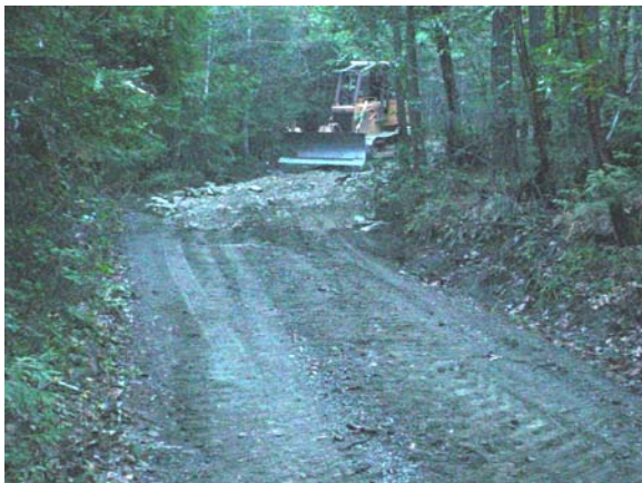
Fig 52. Dozer used to spread rock to outslope the road
