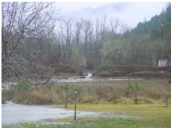
Fig 59. Dam failure with overflow of pond
