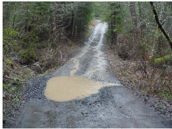
Drainage on roadbed that empties into creek system – Spring Creek driveway
