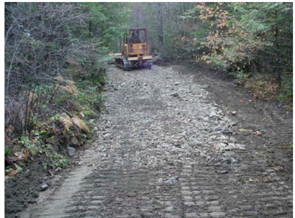
Fig 54. Smoothing and sculpting the road for erosion control
